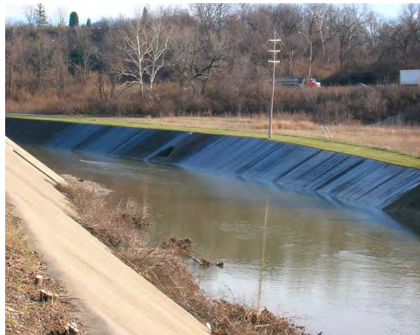
A section of channelized Mill Creek. One can easily imagine returning the banks to a natural edge, creating wetlands to slow stormwater velocity meanwhile naturally treating it before reaching the Creek. Naturally occurring vegetation is currently a maintenance problem for the City but could become part of the solution if allowed to flourish.
