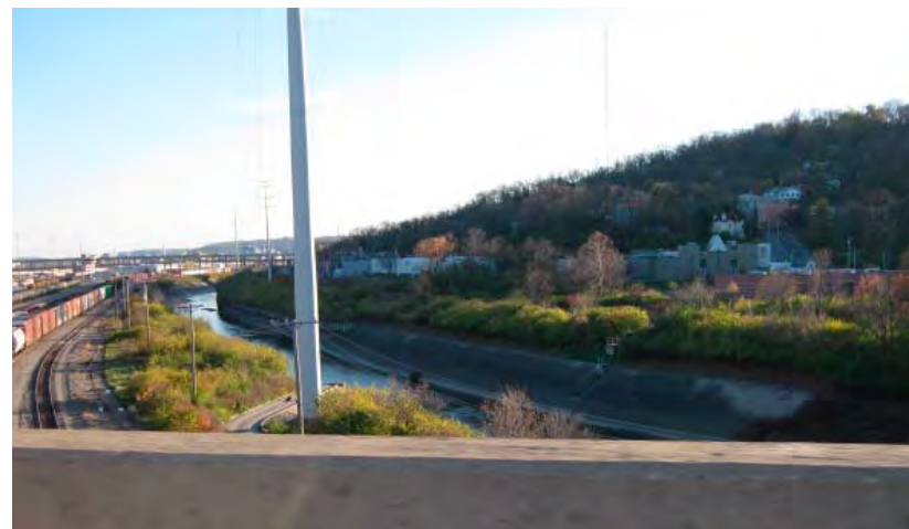
MILL CREEK ALONG THE RAIL YARD
